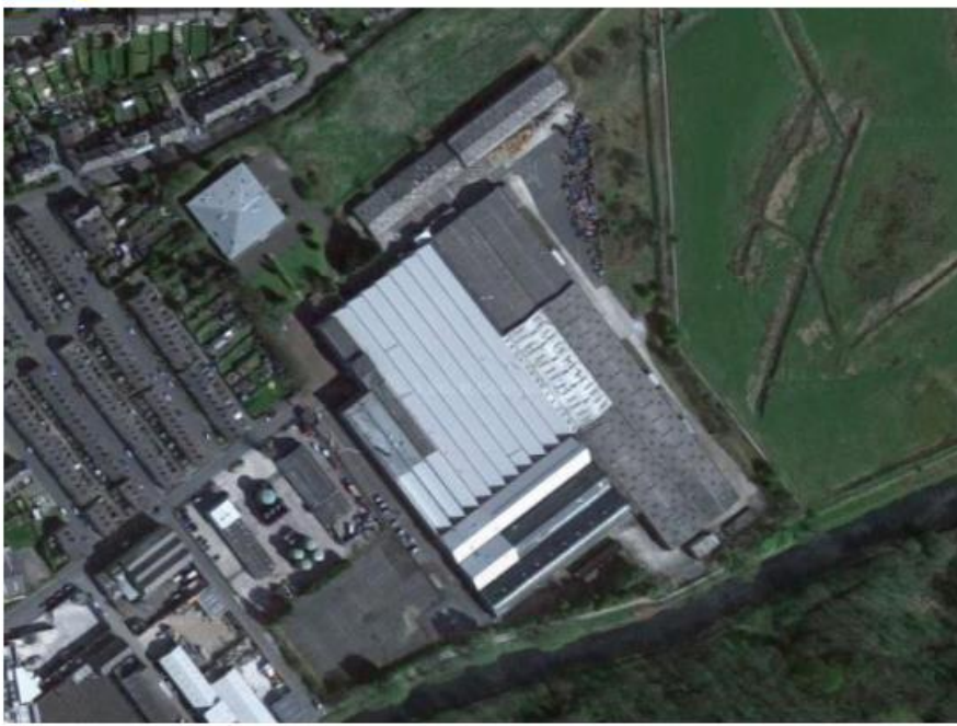
Homes England has already started demolition work on the former factory in Padiham
