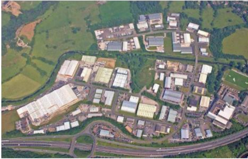
Lomeshaye Industrial Estate
