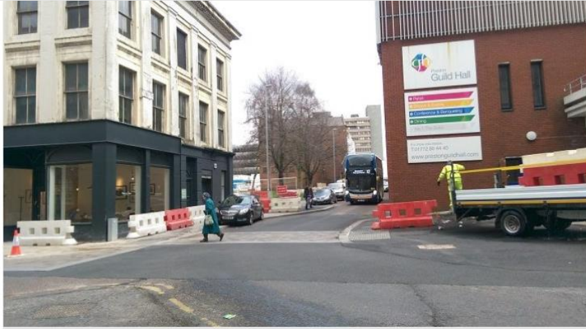
Work continues between Lord Street and Lancaster Road
