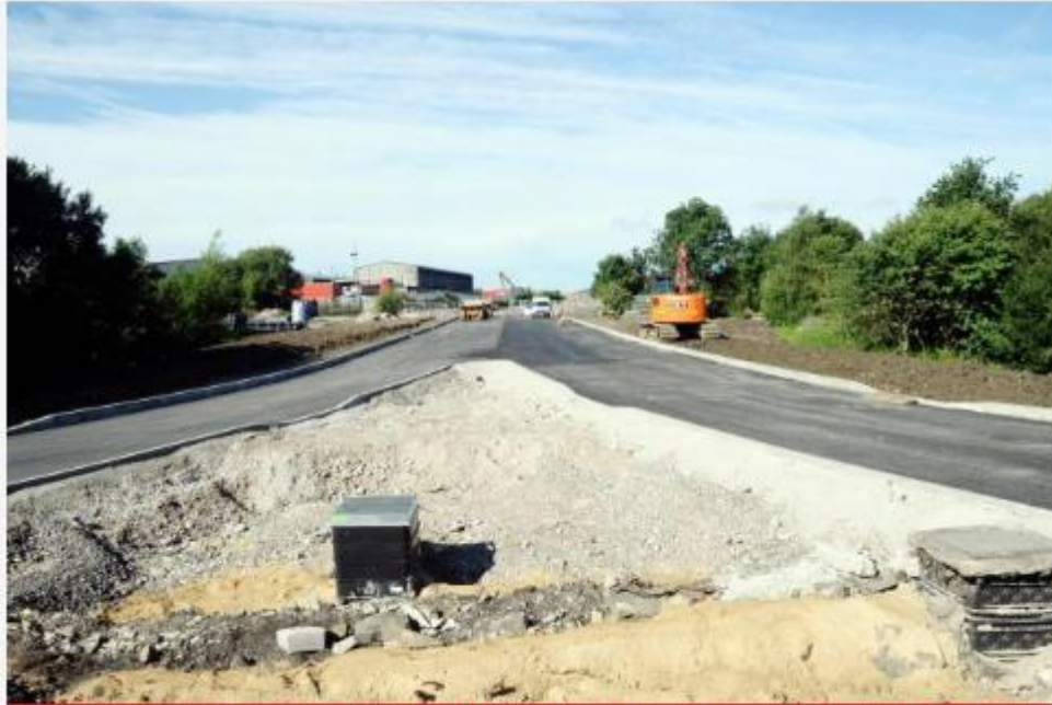
Pennine Reach Development, Blackburn - looking from Whitebirk roundabout
